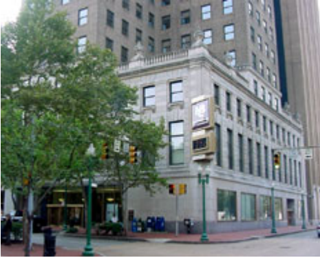
Kanawha Valley Building, 300 Capitol St., Charleston, WV
